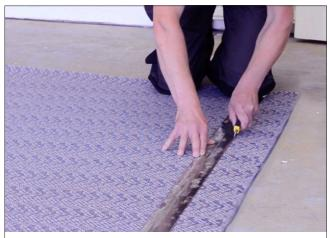
Before gluing: cut the pieces to size with the short ruler (adding spare cm's as overlay) if need be taking the pattern repeat into account.
