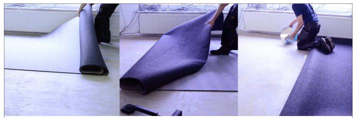
Apply the carpet glue for the first part using the trowel A permanent adhesive system is recommended to fix the carpet directly to a suitably prepared sub-floor.
