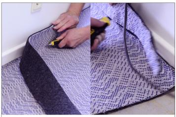
Trim along the wall using the hooked knife. If possible, wait untill the next day till the carpet glue is completely dry. Use the same method for the doors and vent openings.
