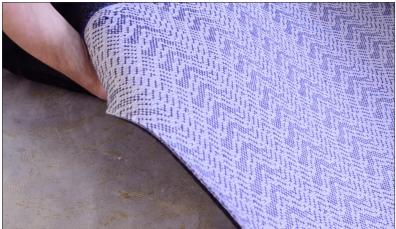
Before starting, decide in which direction the rolls should to be installed. Incoming light and the use of the room can help you with this decision. Note that, according to the woven direction, there's always a more shiny side. If possible, make sure the seams are placed in areas where there is the least traffic.
