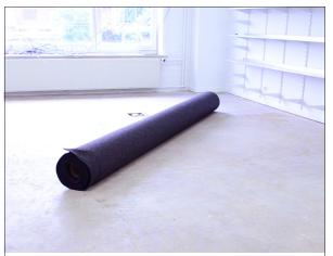
Make sure the surface that will be covered is dry, dust free and smooth. After unwrapping the roll, let it "breathe" in the room it will be fitted for 24 hours (temp.20-22°C, rel. hum. 45-60%).
