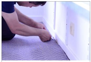
Use the appropriate metal bolster to push the carpet edge slightly between the underside of the skirting and the floor.
