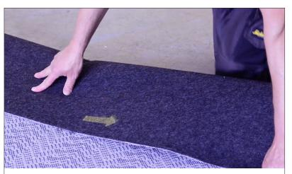
The pieces should all be fitted in the same direction, use the arrows at the back as guidance.
