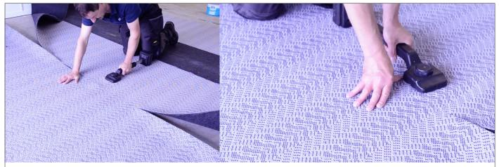
Note: when you kick at one side of the carpet to match the pattern, you should also kick over the whole width of the carpet. This way the carpet is equally stretched. Use the carpet seam roller to ensure the back of the carpet is firmly glued.
