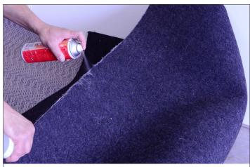
Note : all edges should be concealed with the "anti-fraying spray" before applying the glue for the next part of the installation.
